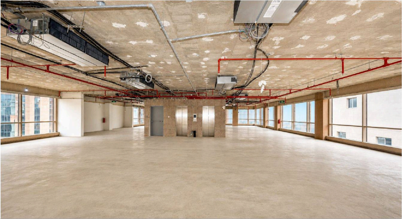
Office floor, current condition
