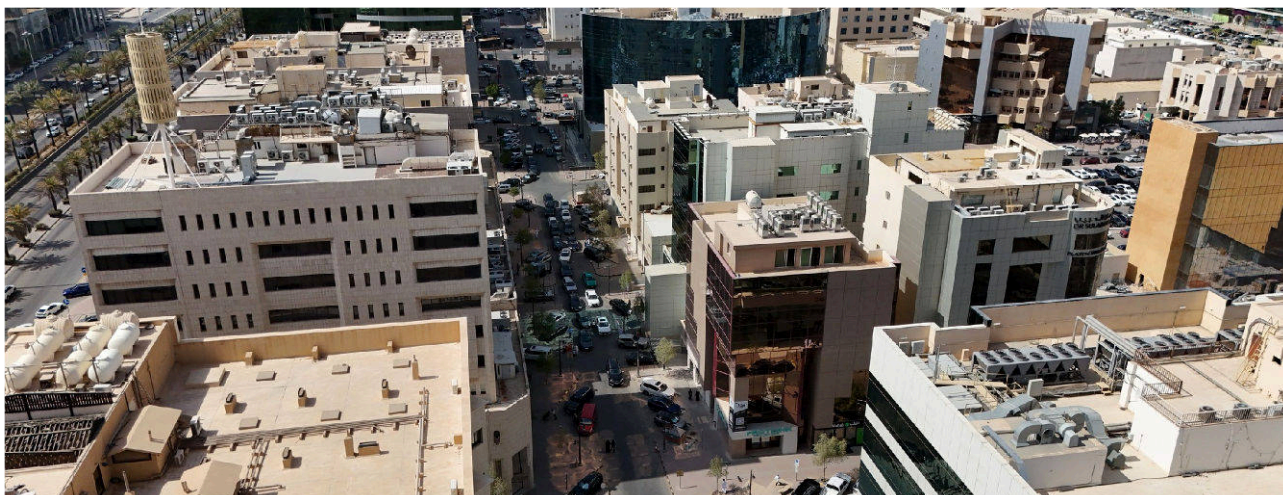
Roof and upper annex from above
